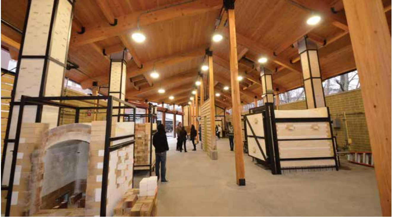
The new outdoor kiln is located behind Harder Hall.
